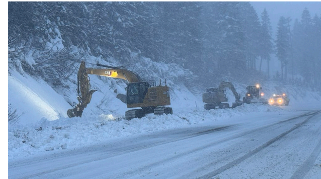
Emergency work underway
