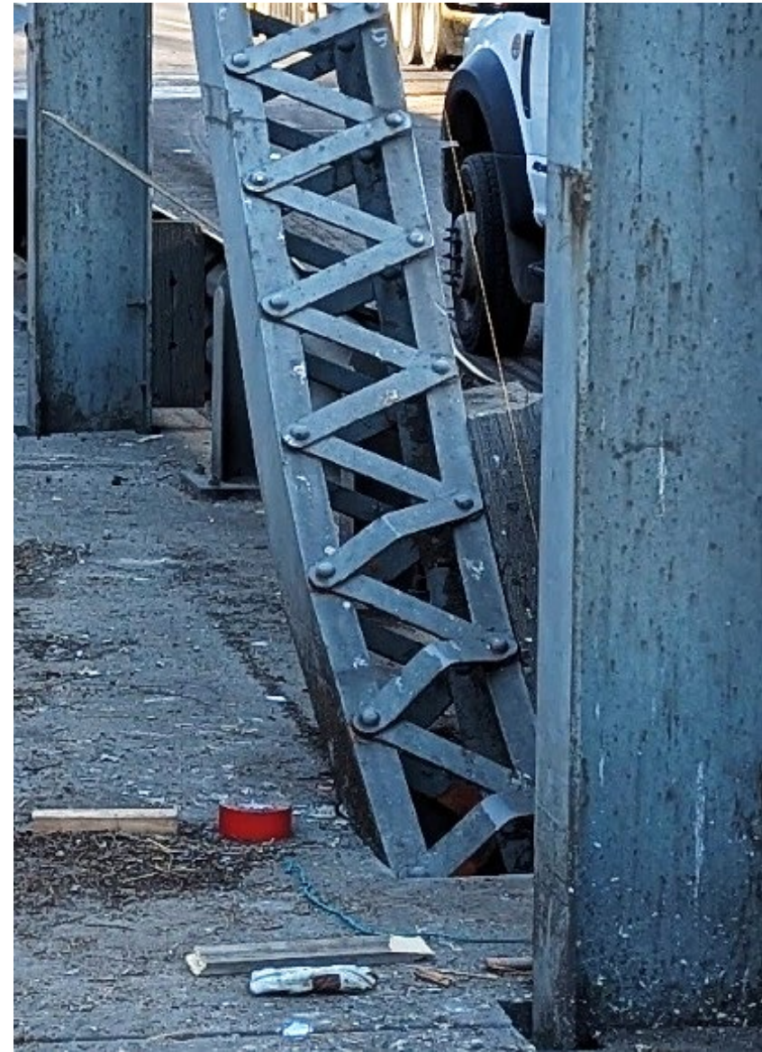
Westbound I-82 Bridge Over Yakima River near Yakima and Selah
