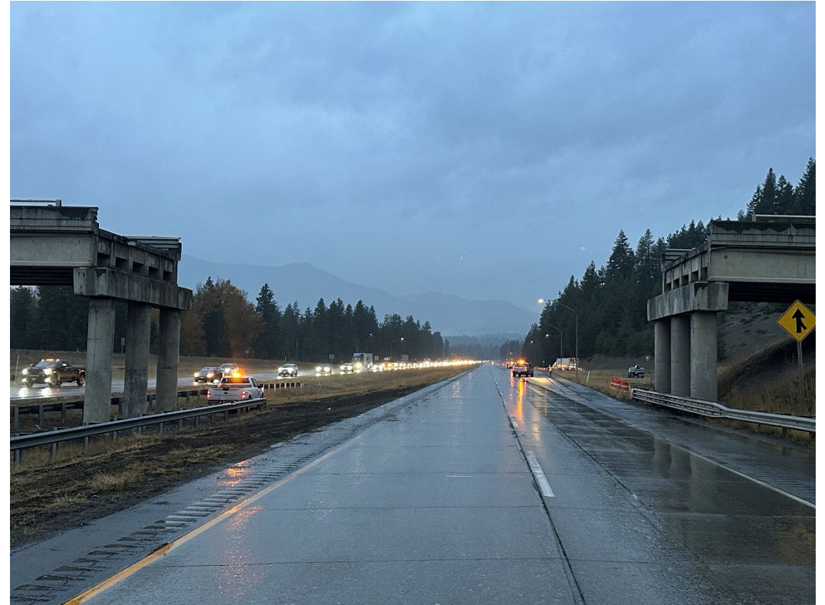
Westbound I-90 open after span demolition.
