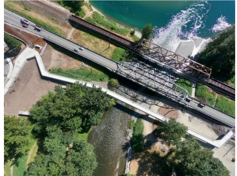
US 2, Sultan Bridge
