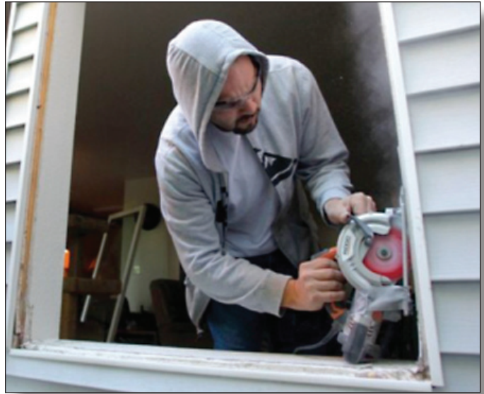
CEEP contractor preparing to install energy efficient windows and weatherstripping.
