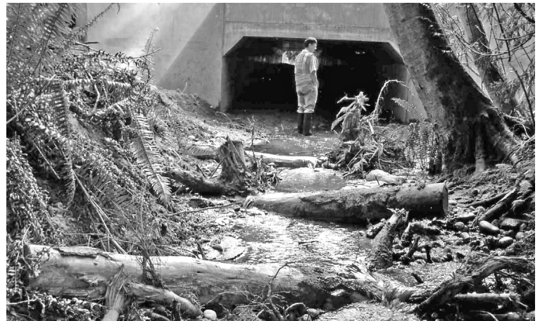
After: A stream simulation design was used at SR 104 to correct the barrier to fish passage.
