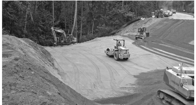
During: Crews backfill and compact soil on top of the newly installed culvert.
