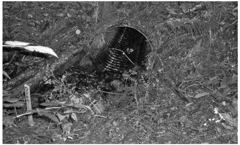
Before: This undersized culvert beneath SR 104 in Jefferson County created a barrier to fish.
