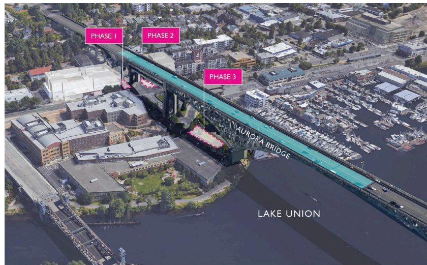
Figure 3. The swales are built adjacent to the Aurora Bridge, a historic structure in Seattle where all five of the region’s salmon species swim to reach the network of rivers and streams for spawning each year. Image credit: Weber Thompson.
