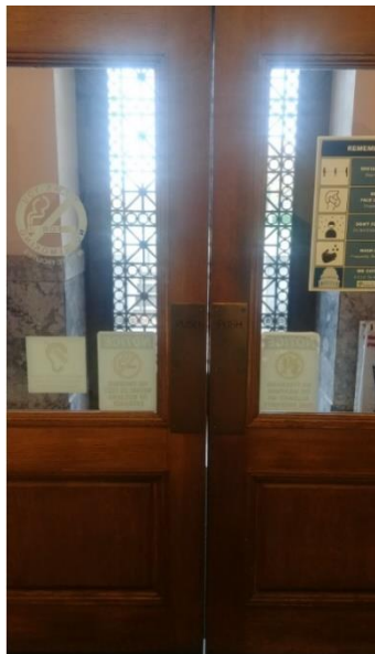
Basement Level Entry Doors
