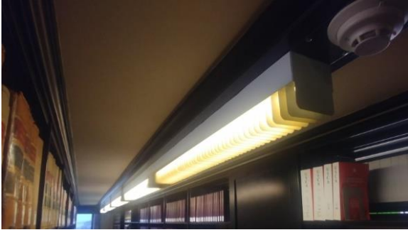
Library T-12 Fluorescent Fixtures installed in 1987
