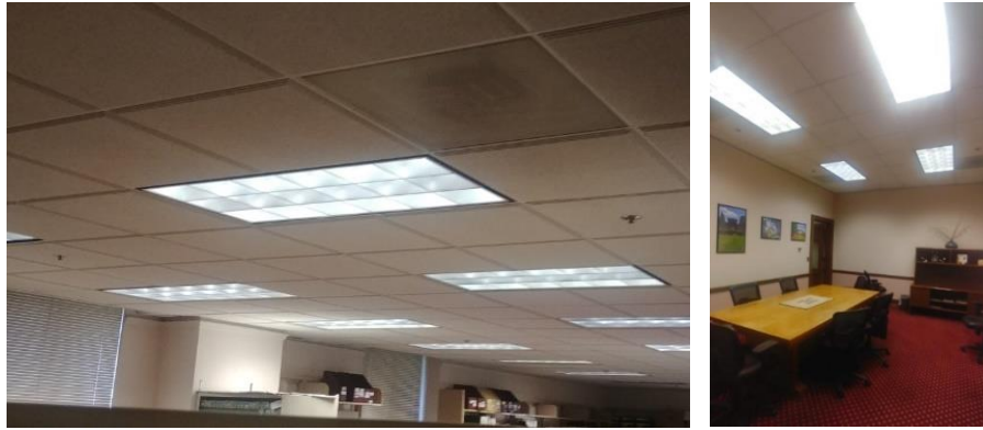
Lower Floor Lighting and a few Conference Spaces – Mostly 2x4 Parabolic Fixtures with T-12 Lamps that were replaced in 1987
