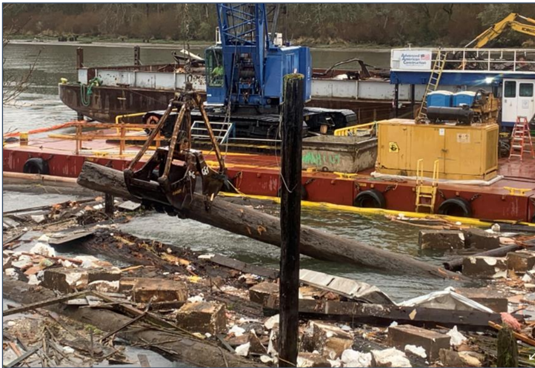
Figure 5. Removal of wood log floatation by clam shell attachment on crane.
