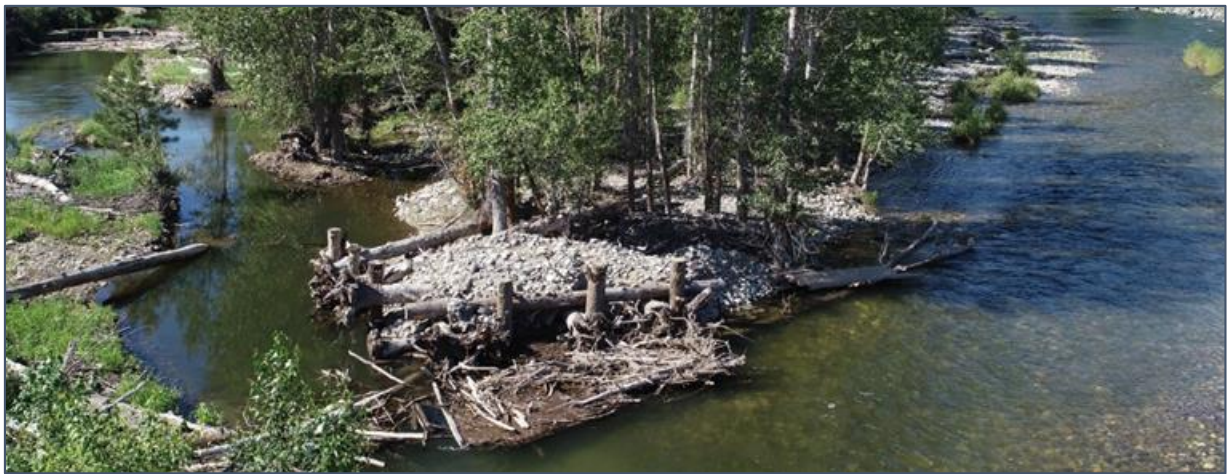
Figure 3. Photo of the installed large woody material and rocks.
