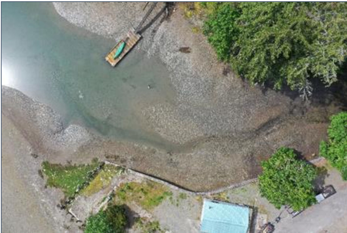
Figure 3. Aerial view of armoring along the creek side of the property.
