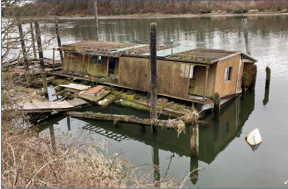
Figure 2. Float house listing into the water 03/29/2023.
