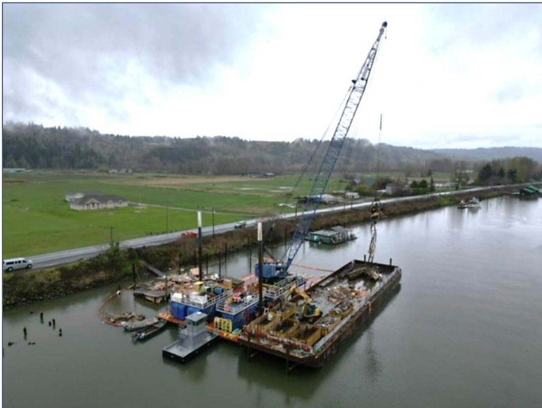
Figure 3. Aerial view of Global's crane and barges, 04/10/2023.
