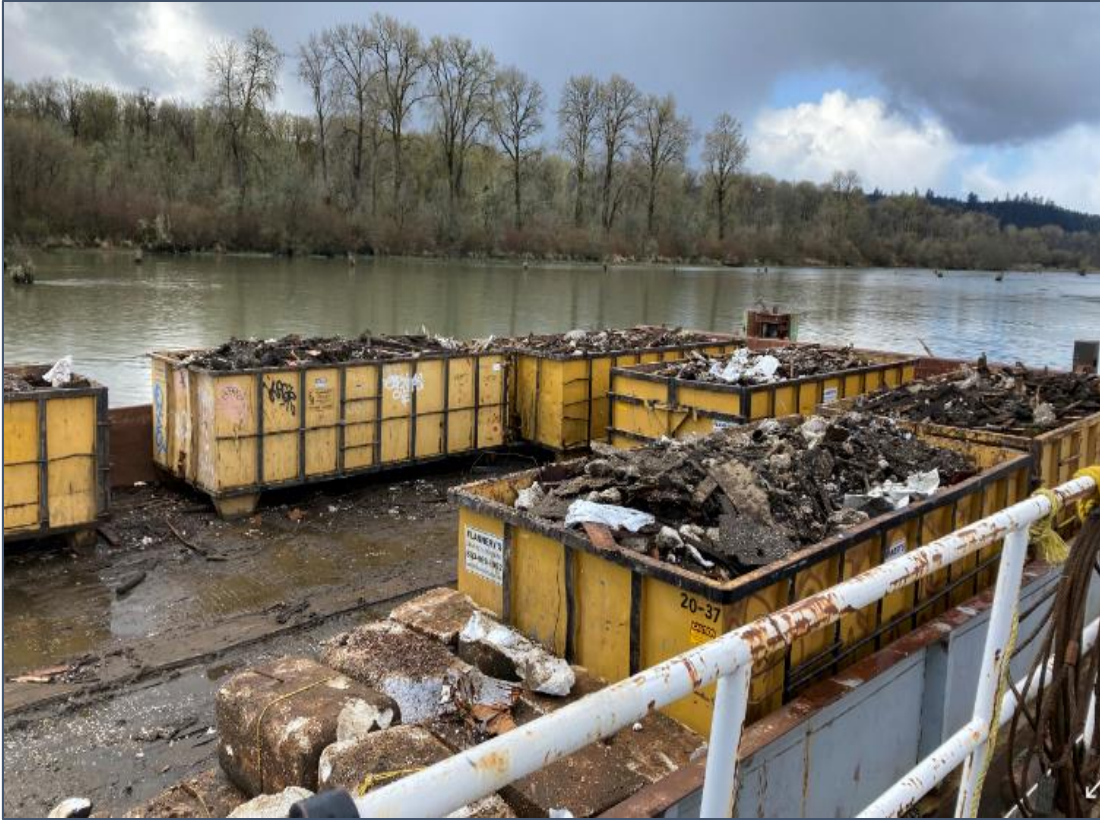
Figure 6. Float house debris in dumpsters on barge, 04/12/2023.
