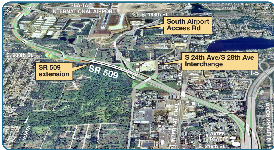
Figure 2-2: aerial view of the I-5/SR 509 Corridor Completion and Freight Improvement Project
