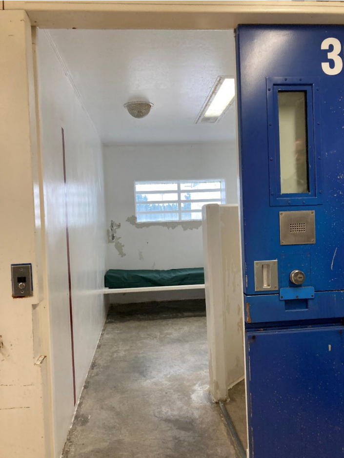
Image 21: Partially renovated solitary confinement cell in MCC-SRTC residential treatment unit.
