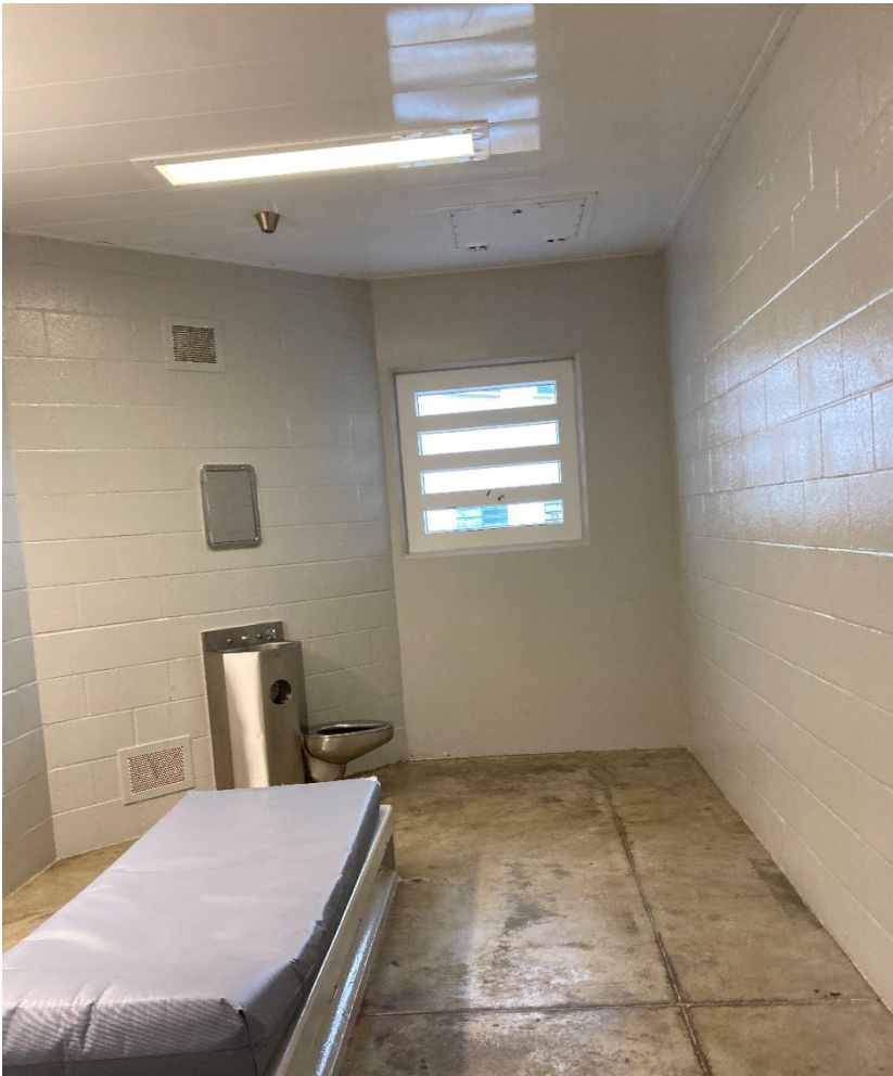
Image 26: Close Observation Area (COA) cell at Monroe Correctional Complex (MCC).
