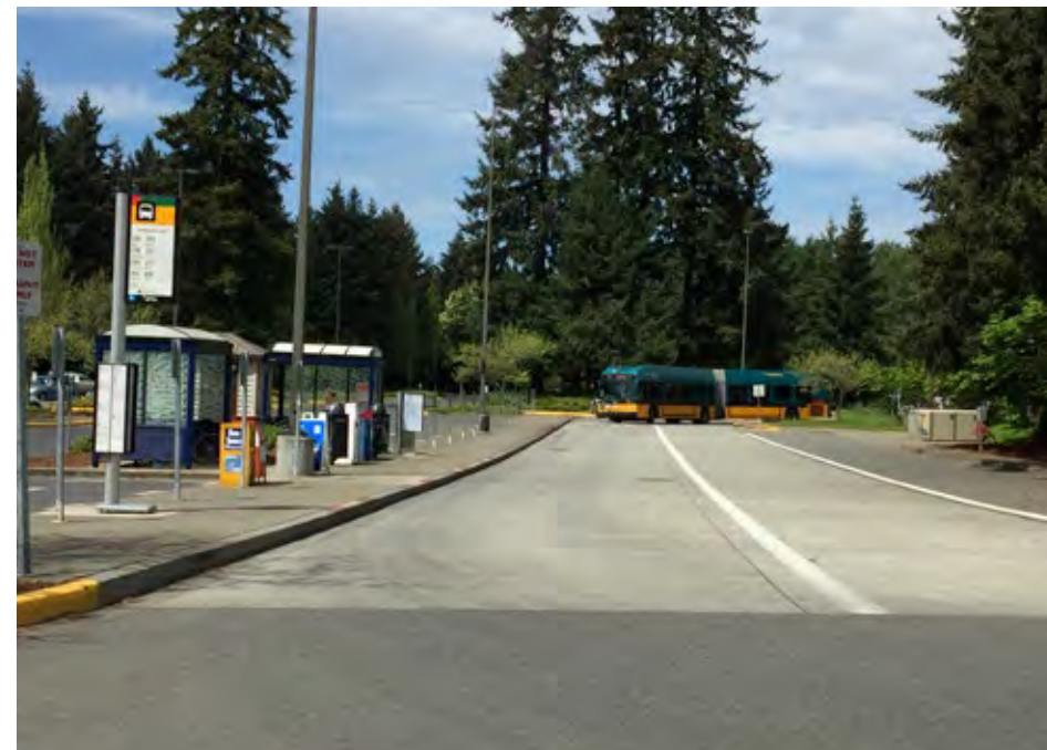
Existing bus service facilities
