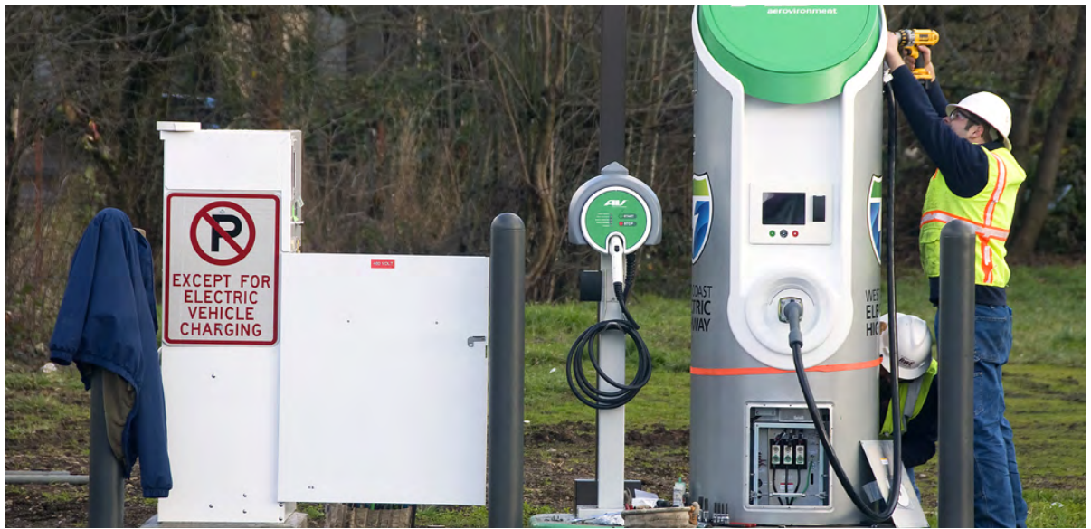
A maintenance technician works on an EV charger.
