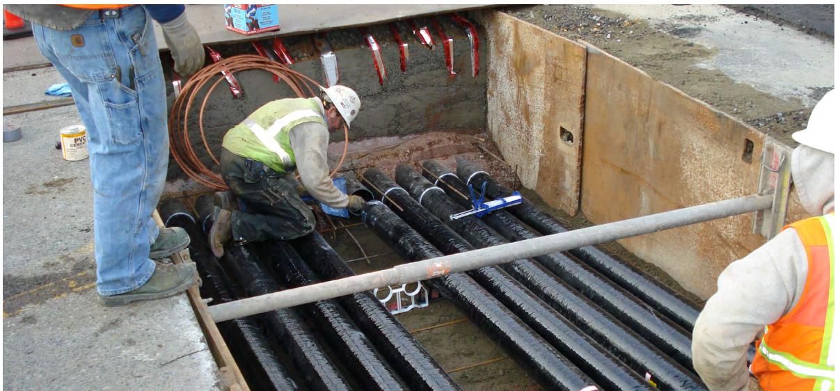
Workers prepare to install EV charging infrastructure in a parking lot.
