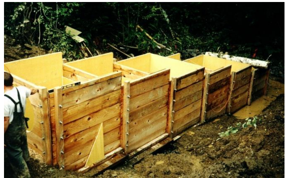
Mason County Fish ladder construction.
