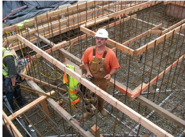
City of Arlington Wastewater treatment plant construction.
