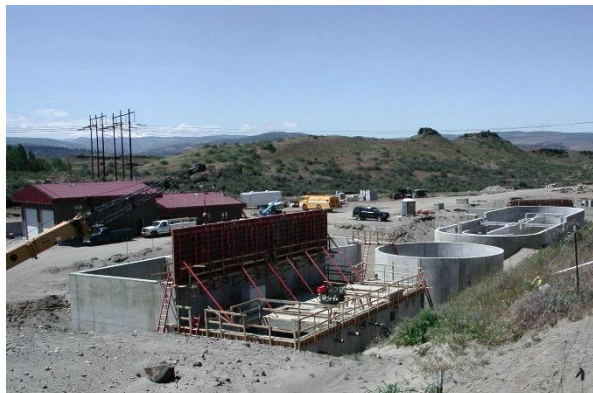
Willapa Bay solid waste facility Site under construction.
