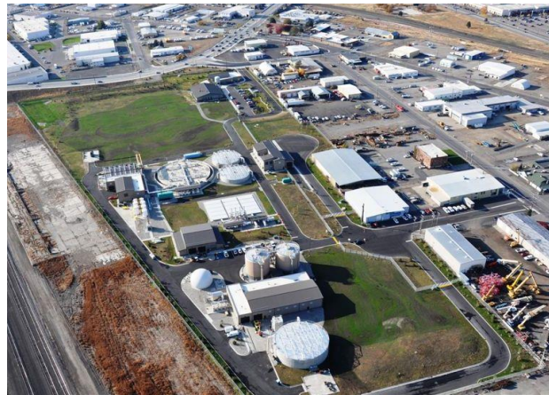
Spokane County Regional Water Reclamation Facility
