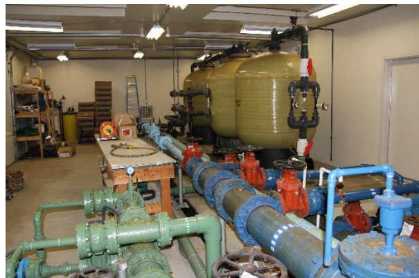
City of Coupeville Water system improvements.
