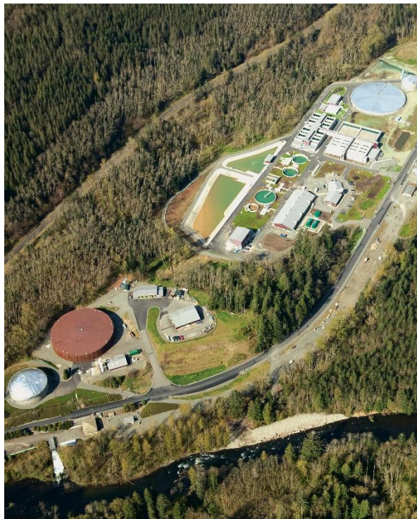
Green River Filtration Facility Miles of pipe connect this plant to its service area.
