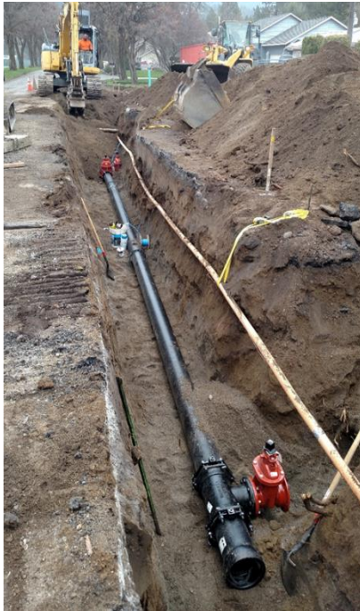
New pipeline construction at the Club.
