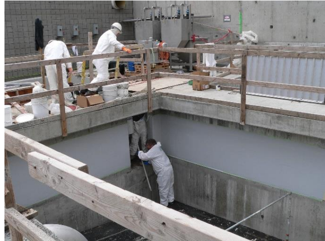
City of Port Orchard Wastewater treatment plant construction.
