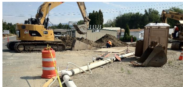
City of Omak Sewer dewatering project site.
