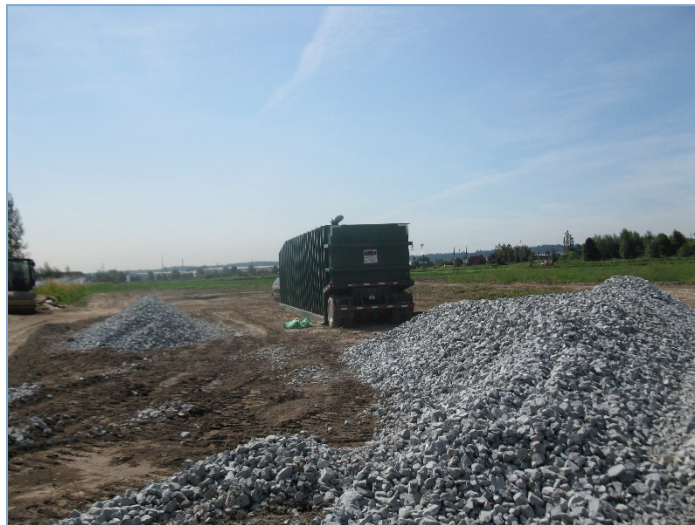
Figure 16: Landfill at the B&L Woodwaste site.
