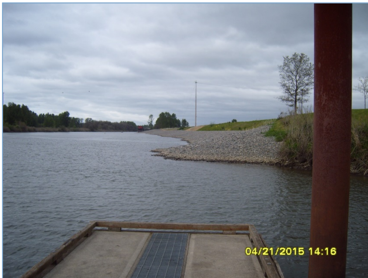
Figure 22: Lake River shore after rehabilitation
