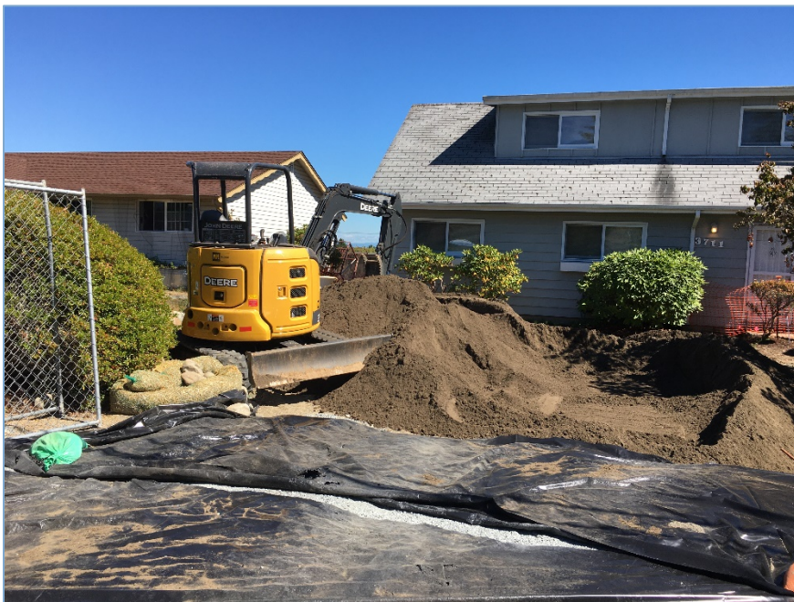
Figure 10: Soil replacement in progress
