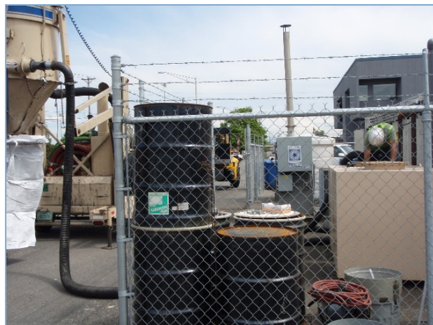
Figure 19: Carbon change out at the former Lilyblad property
