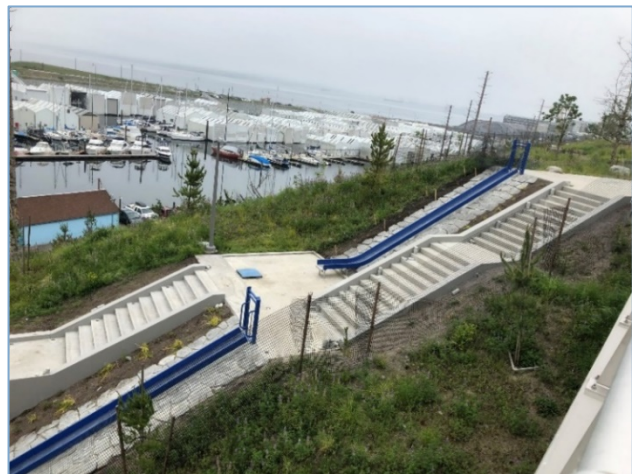
Figure 12: Park slides at Dune Peninsula (Credit: Metro Parks Tacoma).
