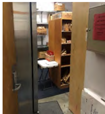
Evidence room – Note Freezer in way of door swing
