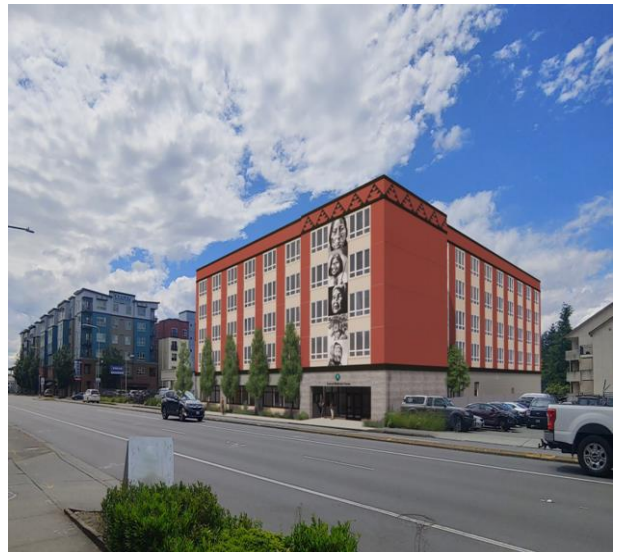
(15) - Sacred Medicine House– 120 units of Permanent Supportive Housing w/ ground floor space for services in North Seattle (Chief Seattle Club) – Scheduled Opening 1 st Quarter 2024
