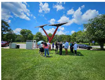
Figure 18: Georgia's first solar-powered photovoltaic for electric vehicle (PV4EV) charging station at The Ray's Visitor Center.
