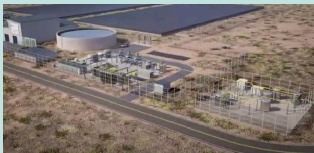
Anaerobic Digesters and RNG Facilities
