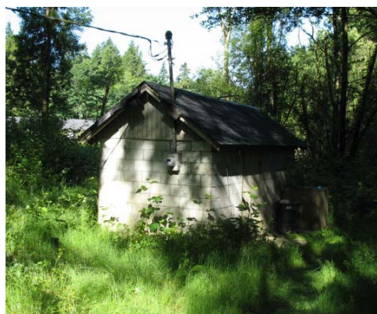
South Keyport Heights Pumphouse
