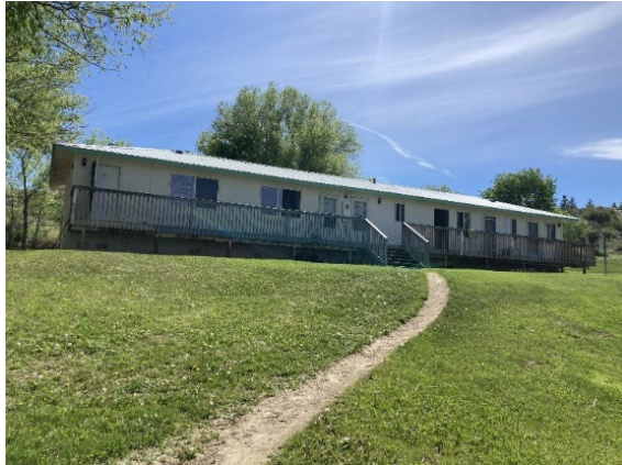
Temporary worker housing inspection Source: ASWS
