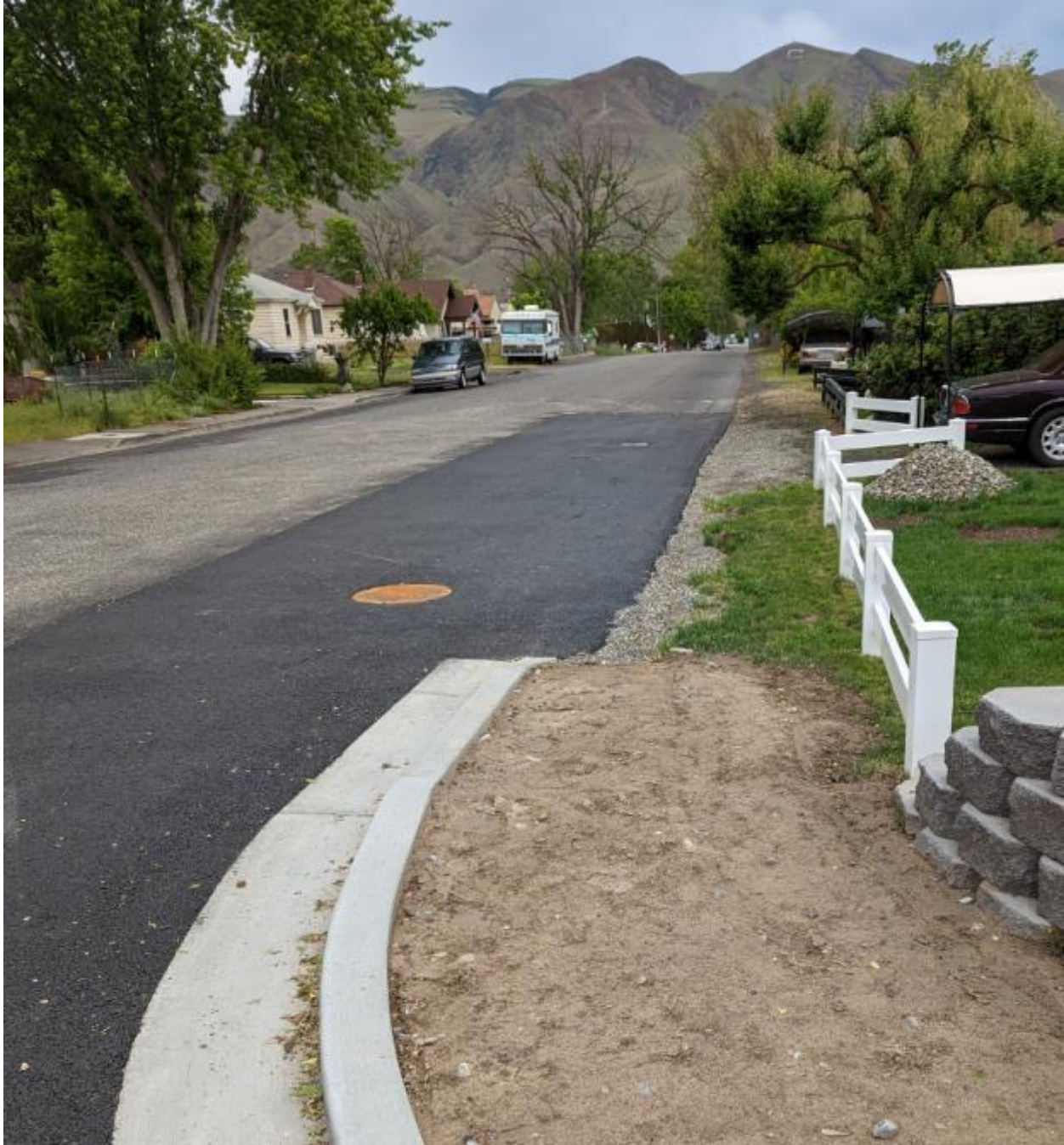
Figure 40: Completed sub-surface infiltration trench with inspection and maintenance ports.
