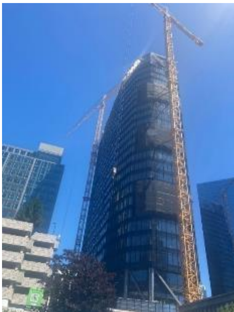
Figure 34: Building development as of July 13 th , 2023. Credit: Ecology
