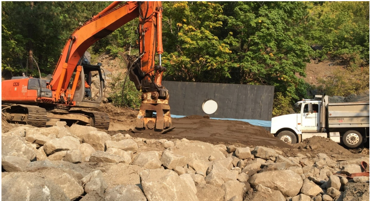
City of Leavenworth Fish screen replacement work near Boulder Field
