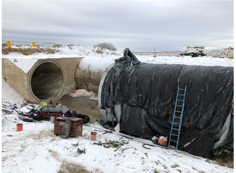
Kansas Prairie 2 siphon construction
