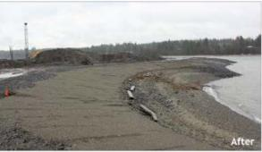
**Photo 17a and b:** More than 8,500 creosote-soaked pilings and 5,600 tons of steel, concrete, and debris were removed from the Port Gamble Bay and Mill cleanup site between 2015 and 2017. As of 2017, shellfish and wildlife are returning to where the sawmill once stood. Photo credit: Ecology (2015, 2017)
