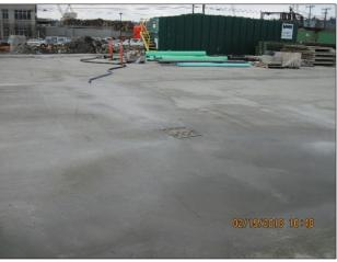
**Photo 30a and b (before and after):** Seattle Iron & Metals Truck Parking showing muddy stormwater (before) and paved surface with stormwater treatment in background (after). Stormwater collection and treatment installed as a result of an Administrative Order. Photo credit: Ecology
