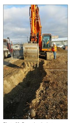
**Photo 20:** Removing the last significant area of PCB contaminated soil at the City Parcel site (CSID 1023) in Spokane. Photo credit: Ecology (2016).
