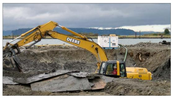
**Photo 37:** Deep-soil excavation helped clean up groundwater impacted by petroleum contamination at the West End site on Everett's waterfront. Photo credit: Ecology (2007).
