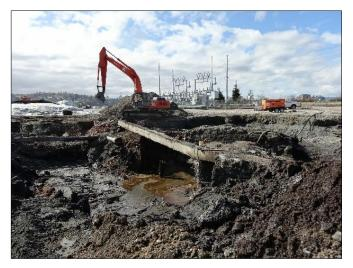
Photo 1: Petroleum-contaminated soil and groundwater are removed as part of an upland interim action at the former Kimberly-Clark Worldwide pulp and paper mill, Everett waterfront, March 2014. Photo credit: Department of Ecology.
