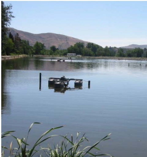
Current unlined lagoons are not meeting TMDL limits for phosphorus, one of its many problems. Ecology Photo
