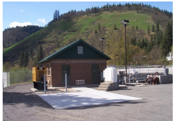
Klickitat community's new wastewater treatment plant up and running. Ecology photo
