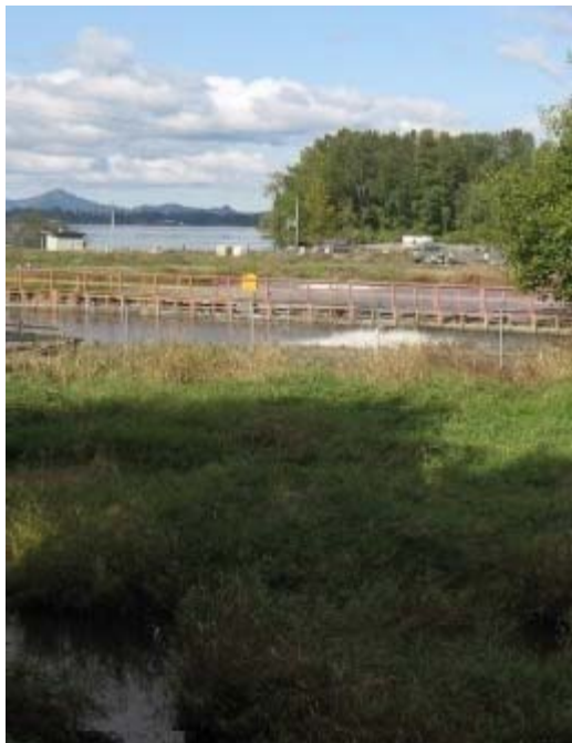
Cathlamet's existing unlined sewage stabilization lagoons are sandwiched in between the wetland (foreground) and the Columbia River (background).
