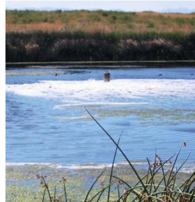
Current lagoons are leaking into ground water, causing need for an upgrade. Ecology photo
