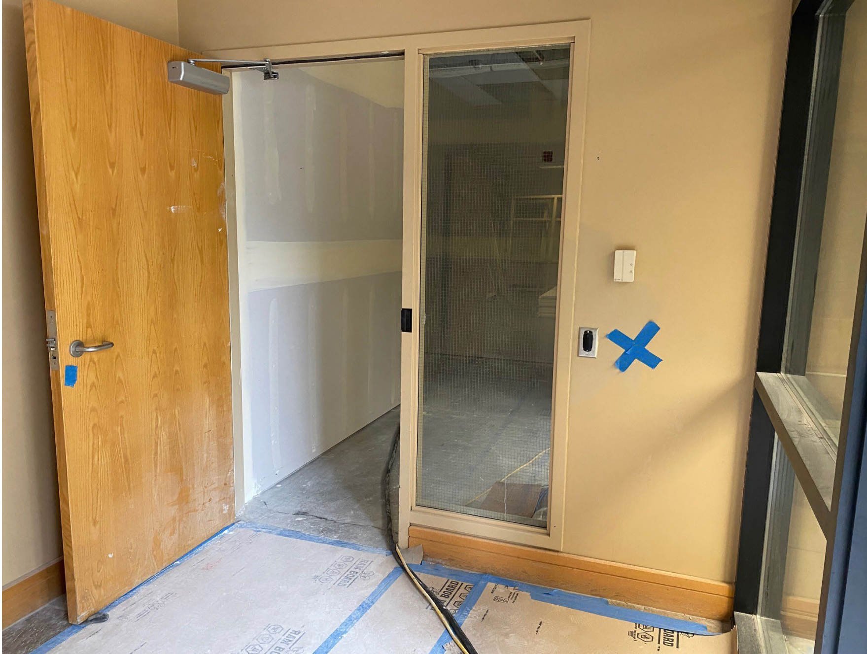
Federal Way Tox Lab – Evidence Drop-Off @ South Entrance
