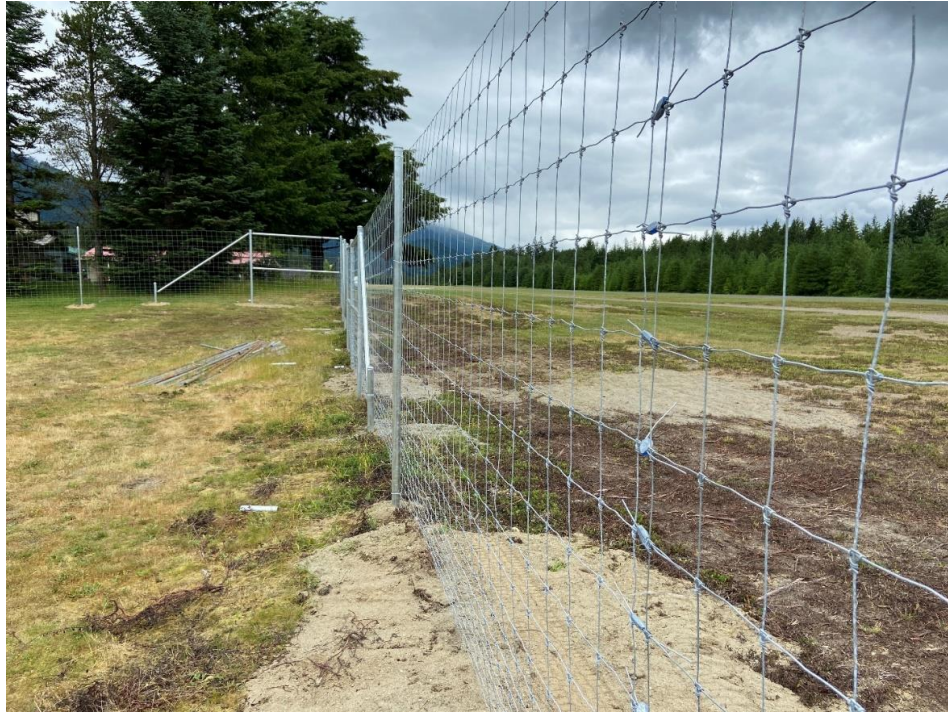
Detail of the New Zealand style fence installed along the school's perimeter.
