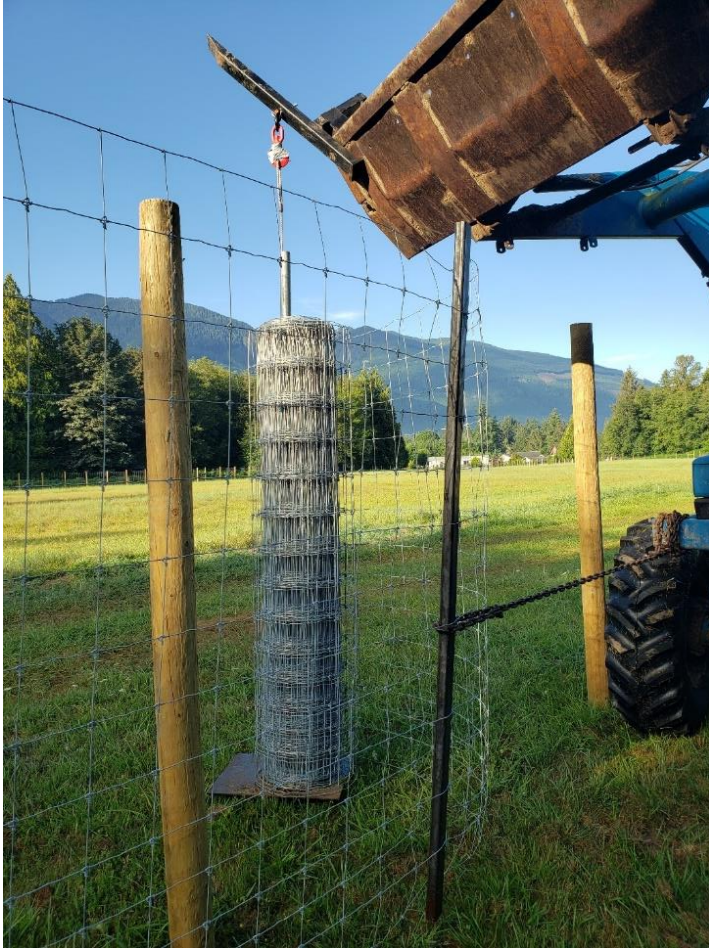
Install of New Zealand style elk fencing along hay pasture boundary.
