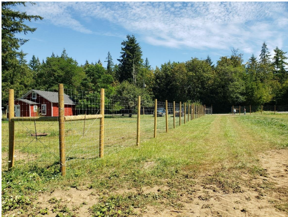
New Zealand style elk fencing installed along the perimeter of a 20-acre hay pasture near SR20.
