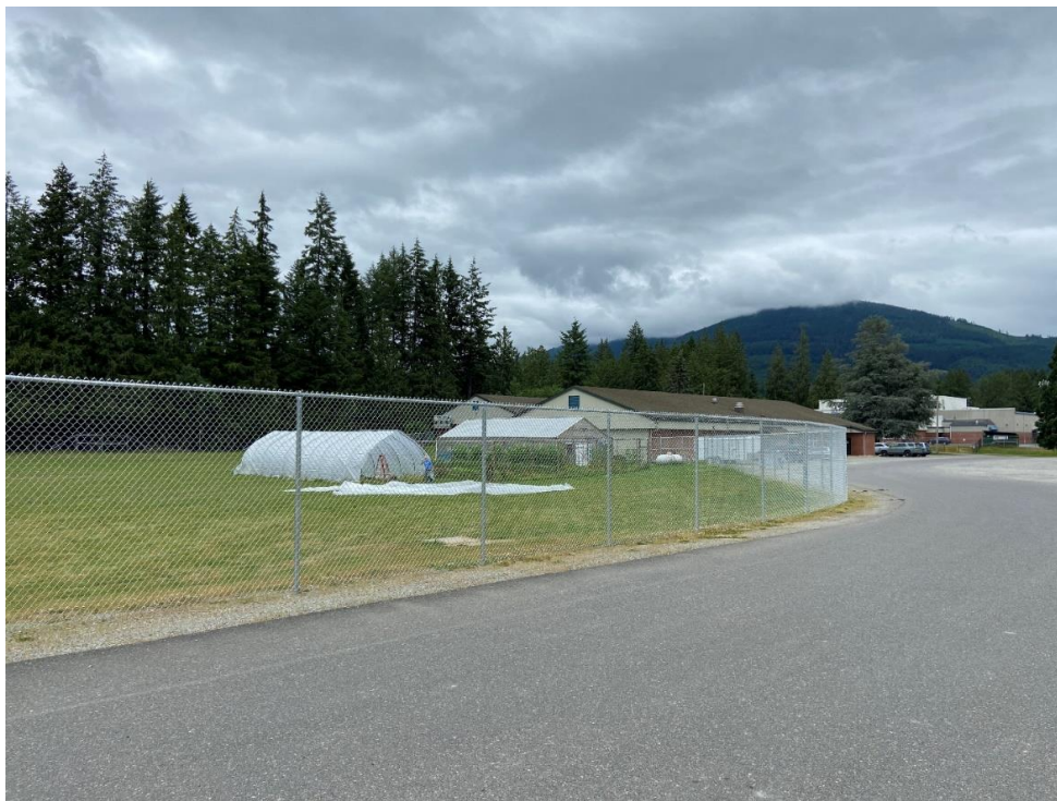
Chain link fence installed around one of the school's recreation fields. The school's greenhouse is in the center of the photo.
