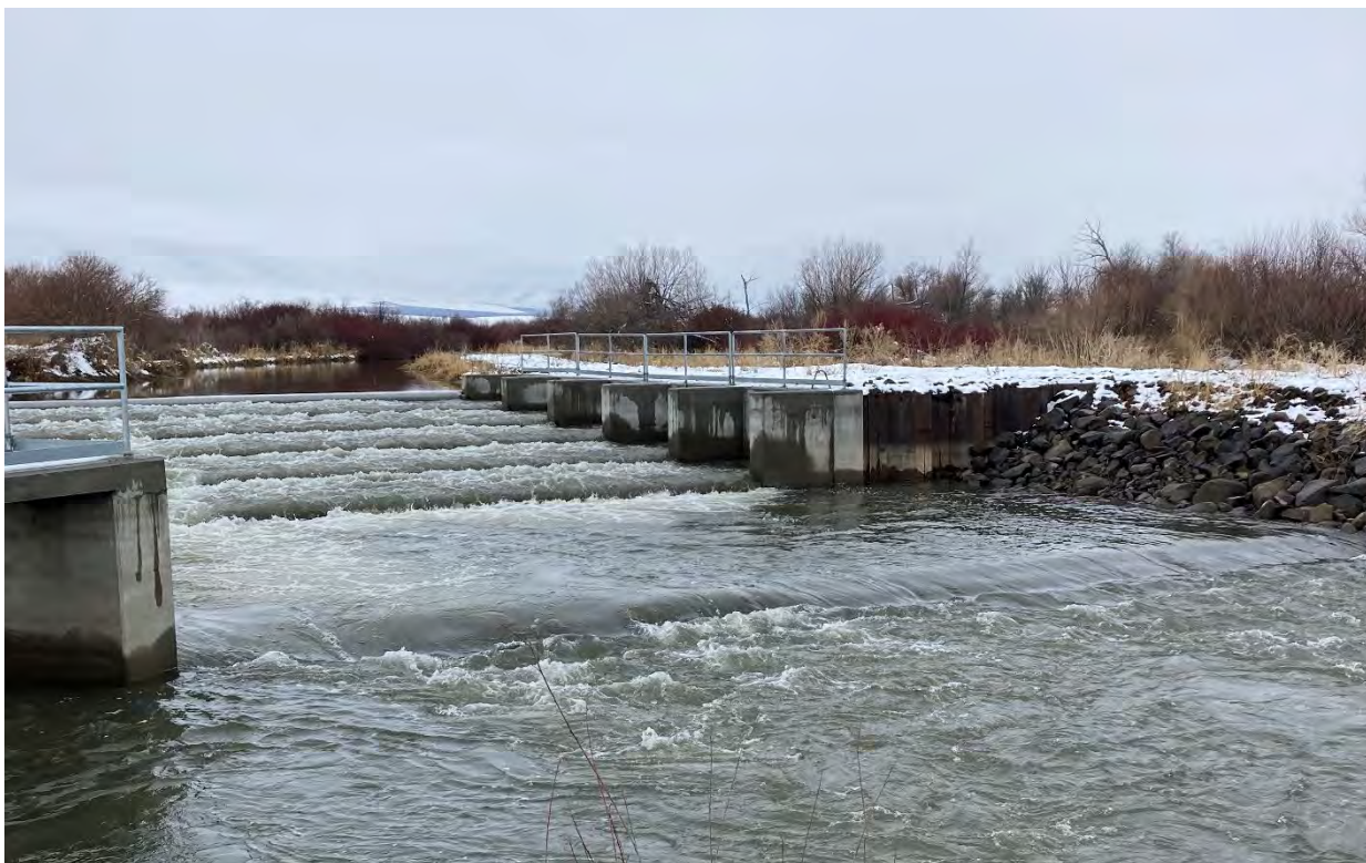
Completed Unit 2 diversion dam rebuild
