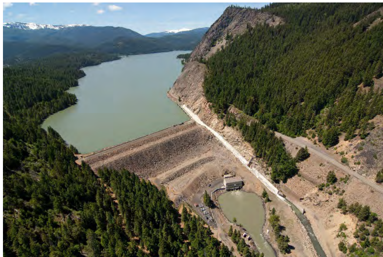
Aerial view of Tieton Dam
