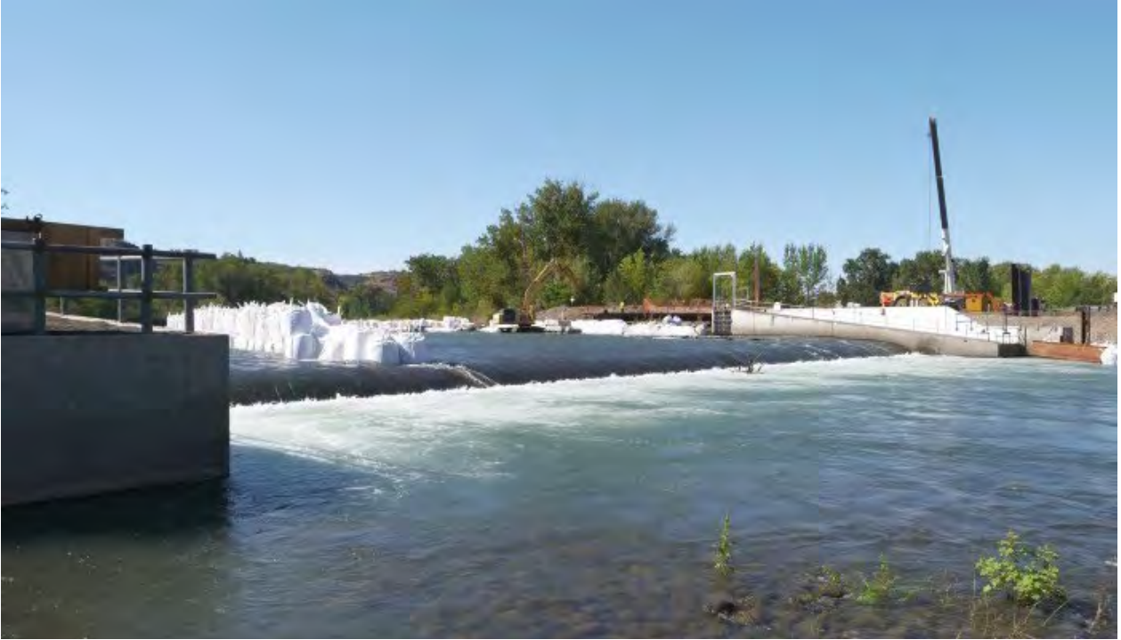
Construction on the Nelson Dam removal project, Naches River.
