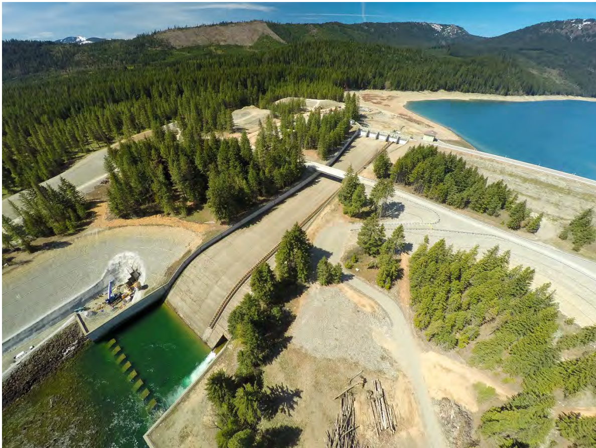
Start of construction, Cle Elum Fish Passage project
