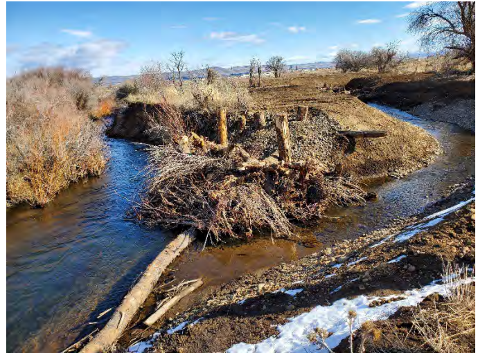
Simcoe Creek large wood floodplain restoration, Yakama Nation Reservation.
