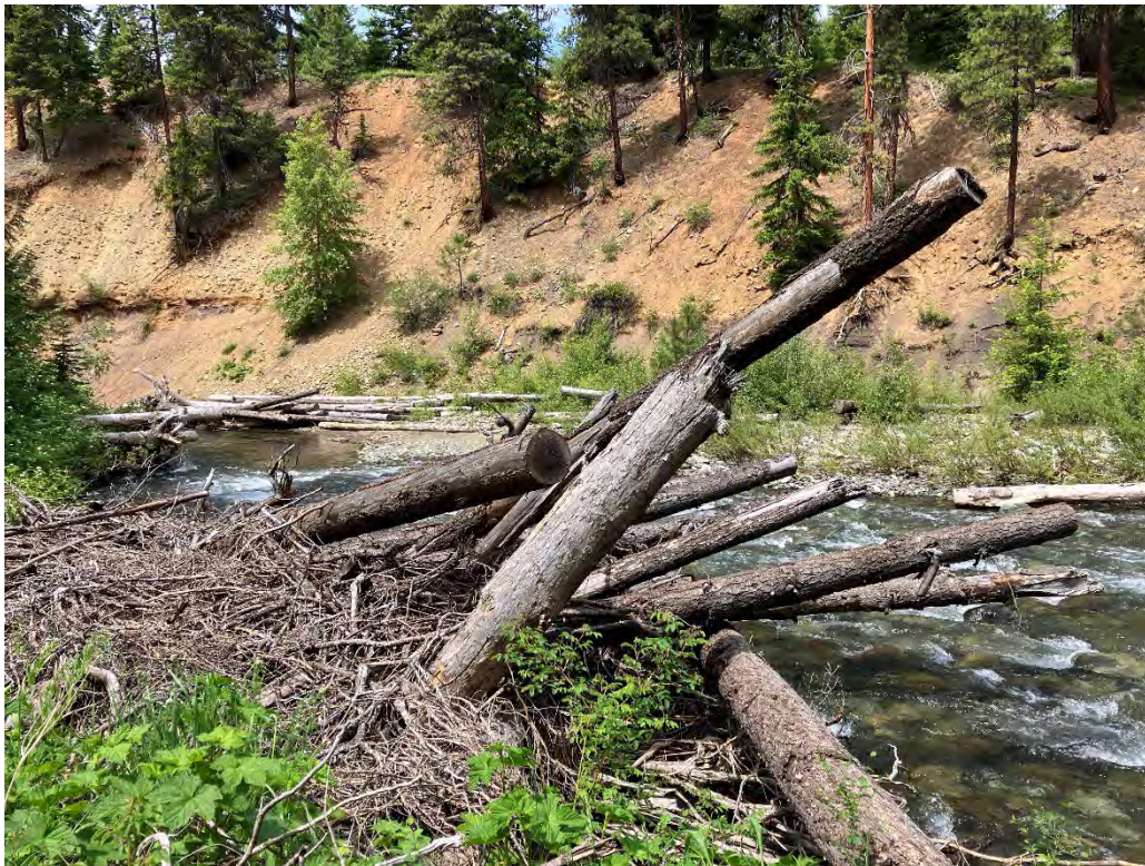
Completed work on the North Fork Teanaway River.
