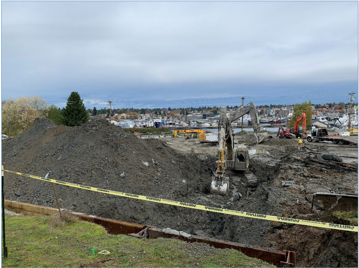
Figure 5: Site cleanup activities underway in 2021
