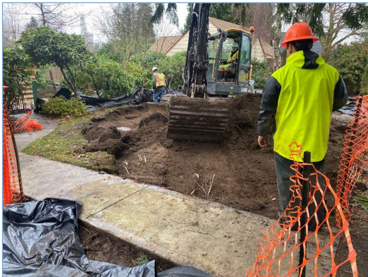
Figure 9: Soil replacement in progress
