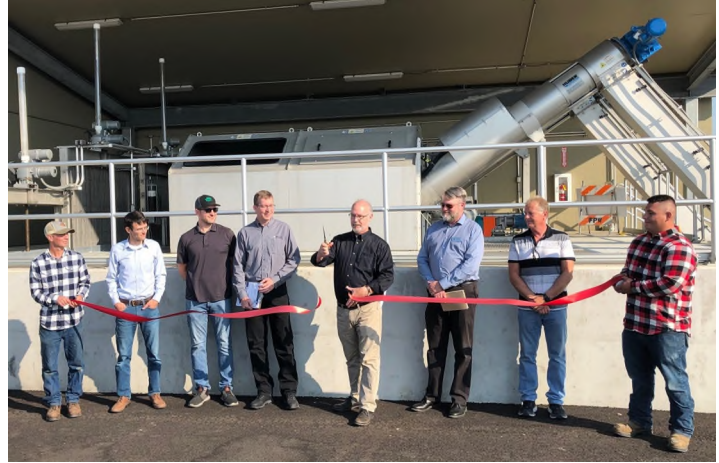
City of Ferndale wastewater treatment plant upgrade, 2022.
