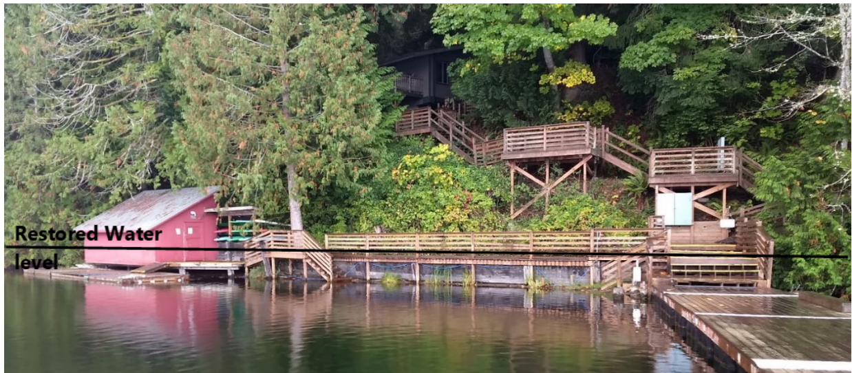
Figure ES-1. Gangway, Decking, and Access Stairs Will Need to be Rebuilt to Accommodate Restored Water Level.
