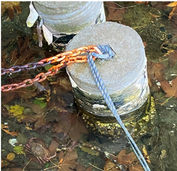
Figure 11. Existing Cement Anchors for Docks in Whiteman Cove.
