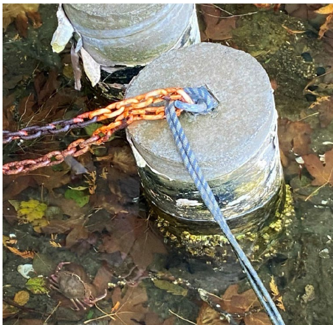
Figure ES-2. Existing Concrete Anchors Used to Secure the Lagoon Dock.
