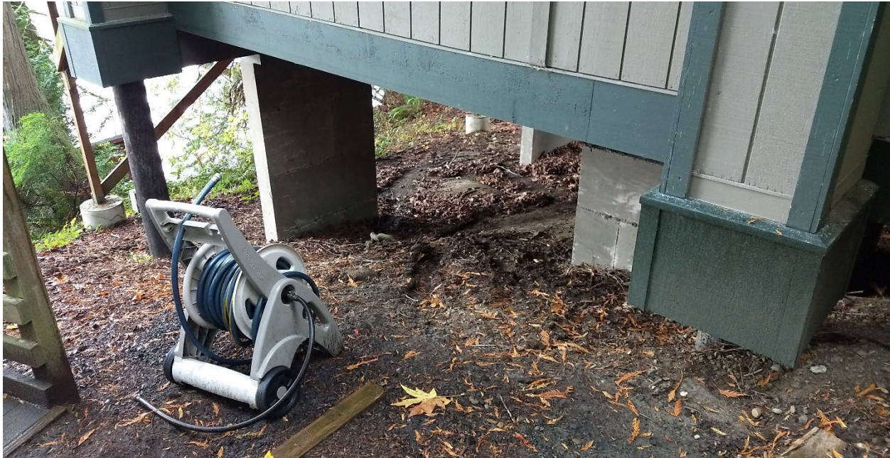
Figure 13. Rills from stormwater Flowing Down the Uplands to the Bluff Face.
