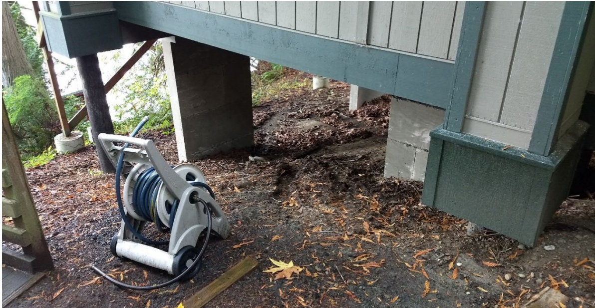
Figure 9. Rills from Stormwater Flowing Down the Uplands to the Bluff Face.
