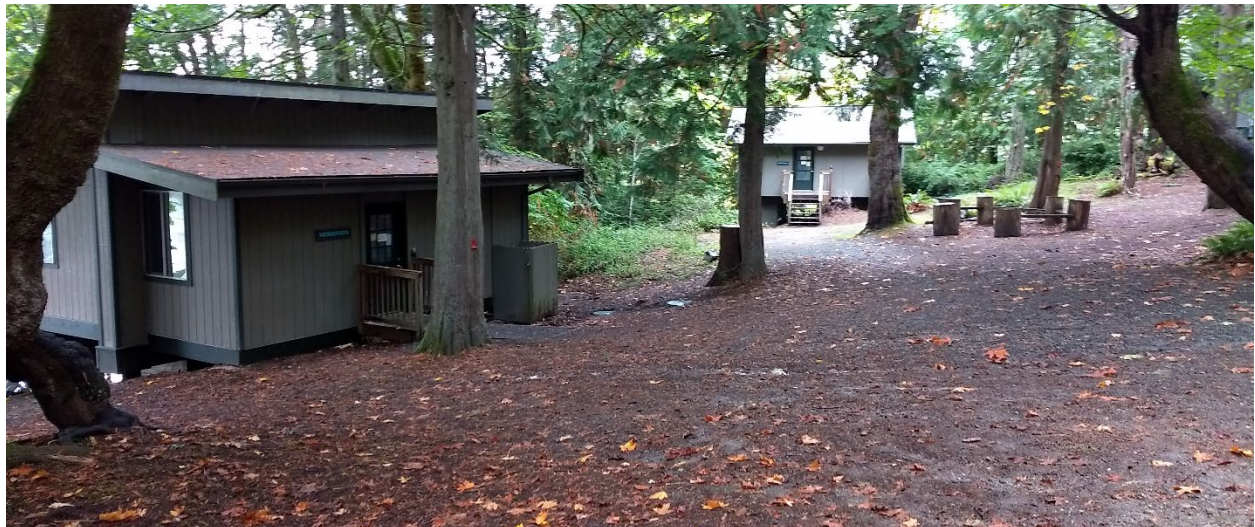
Figure 4. Henderson and Rotary Cabins Near the Bluff Crest.
