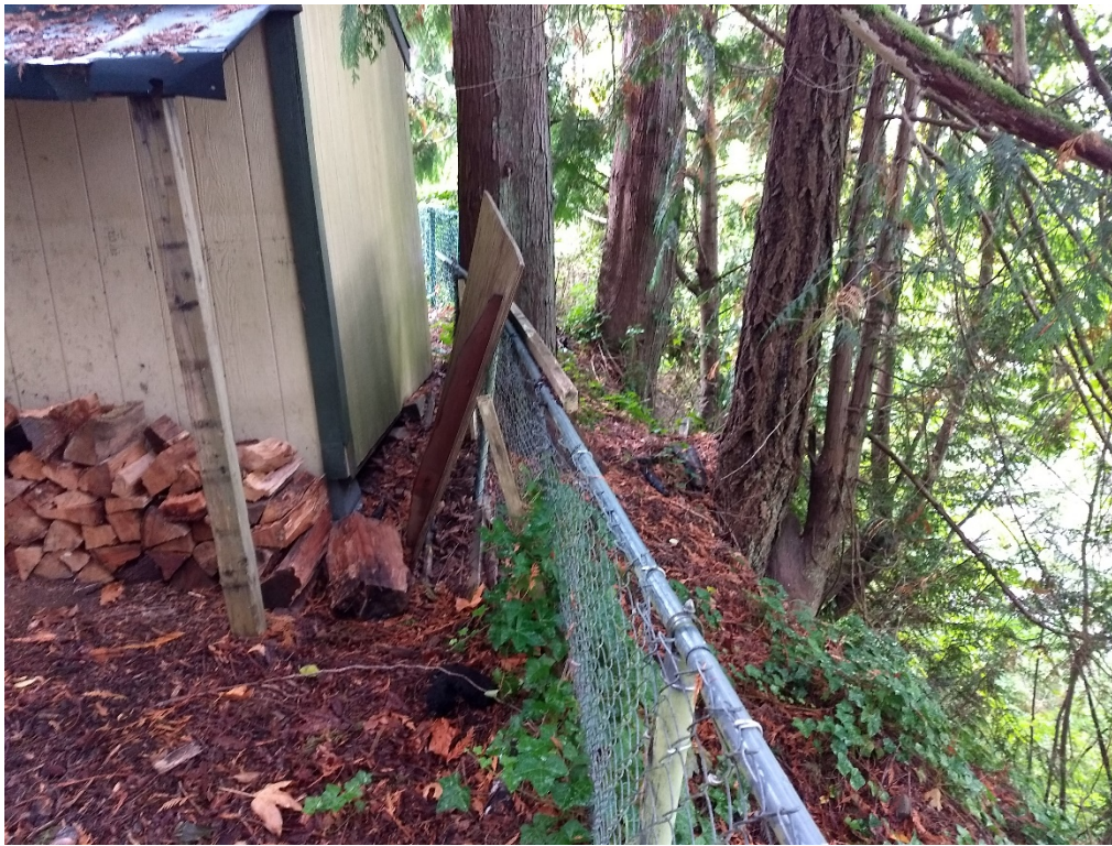
Figure 15. Close Proximity of Storage Shed to Bluff Crest.
