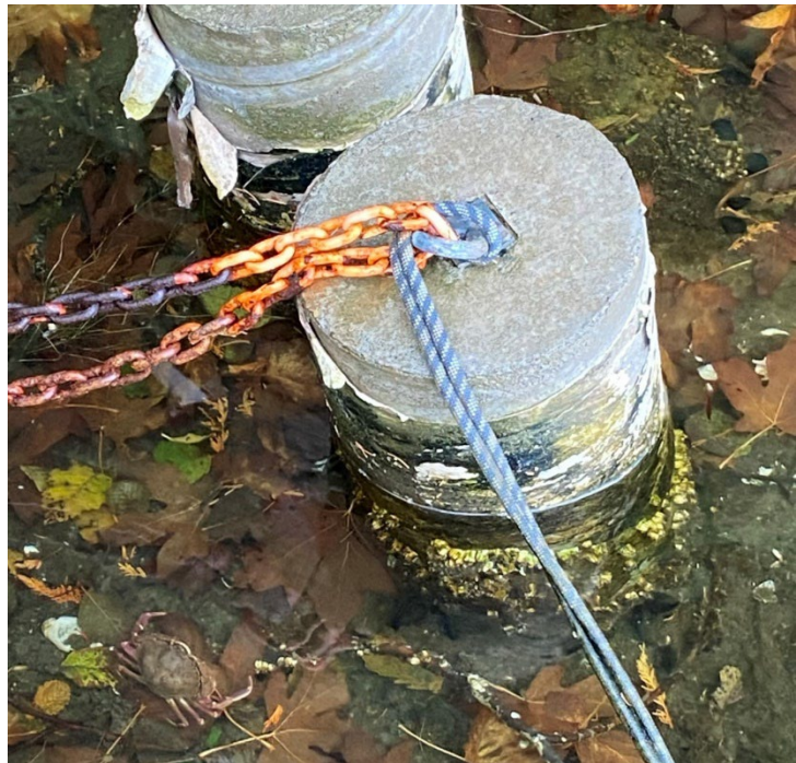
Figure 10. Existing Concrete Anchors Used to Secure the Lagoon Dock.
