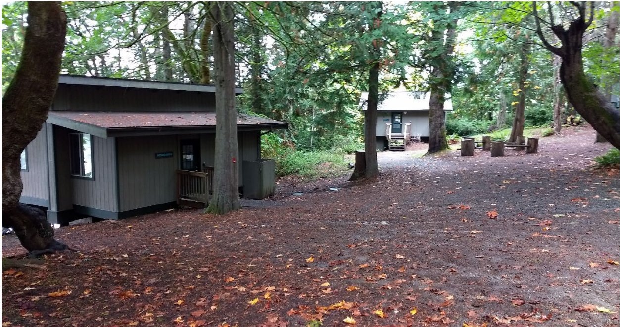
Figure 14. Henderson and Rotary Cabins in Close Proximity to the Bluff Crest.
