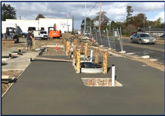
Concrete pad installed after the old tanks were removed and decommissioned.
