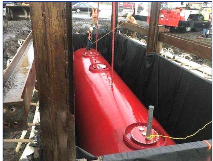
Installation of new multi-chambered UST. Photo credit: Vertex.
