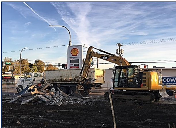
Removing concrete above USTs. Photo credit: Vertex.
