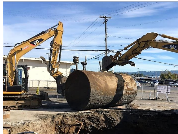
Removed diesel tank. Photo credit: Vertex.
